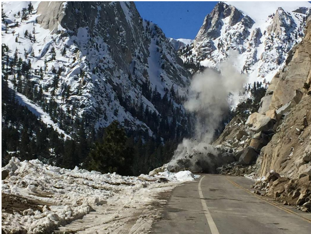
FIGURE 3: WHITNEY PORTAL ROAD ROCKFALL, 2017
