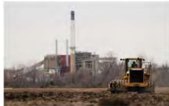
A worker prepares a plot of land for an artificial intelligence data center that works as a virtual power plant being established by private administrator the facility in the Wisconsin Independent Wisconsin | Charles Kandel/AP
