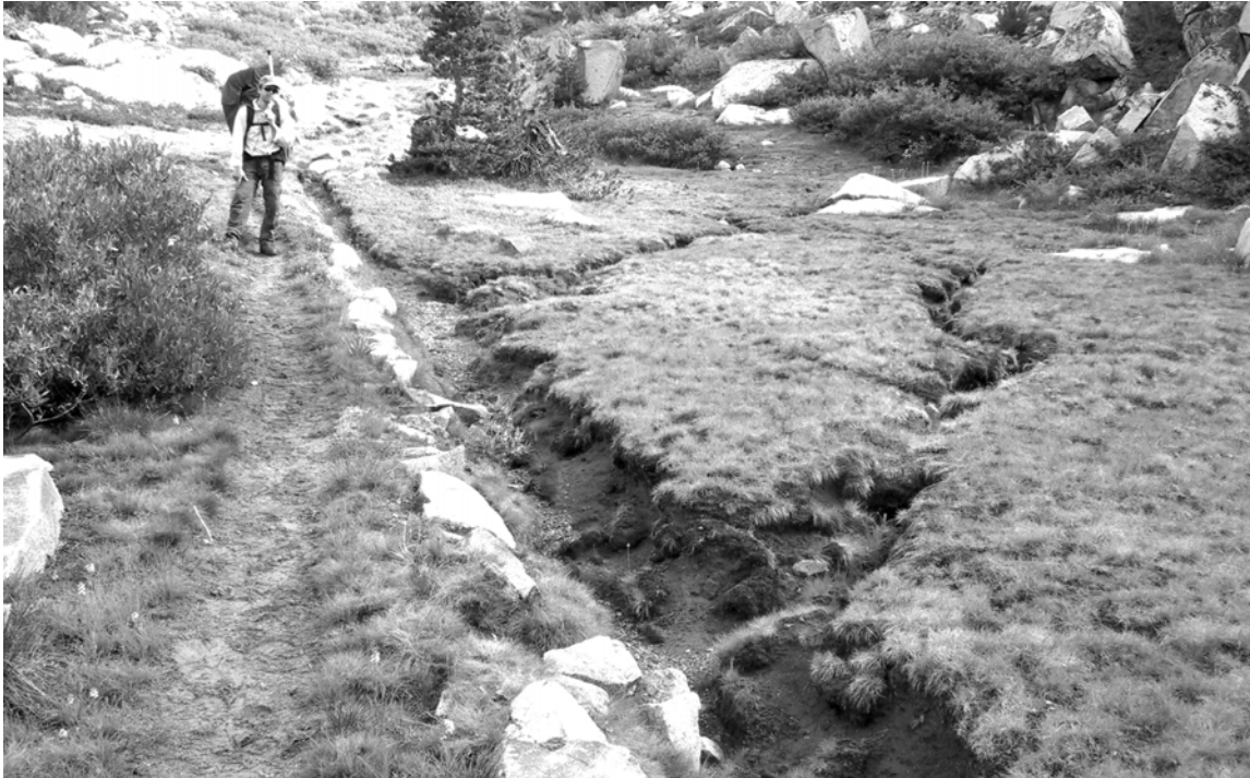
Pacific Crest Trail, south of Seldon Pass. Abandoned, impassable trail and newly developed trail. The old trail on the right captured water from the meadow and uptrail, causing the trail to incise and headcuts to propagate into meadow. The headcuts, shown on the right side of the photo caused loss of productive soil and likely locally lowered the meadow's water table.
