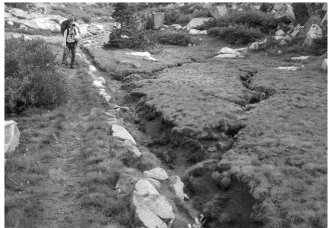
Poor trail alignment and inadequate development, combined with moderate risk factors has led to long-term off-trail impacts, incision, headcutting and meadow damage on this primary system trail
